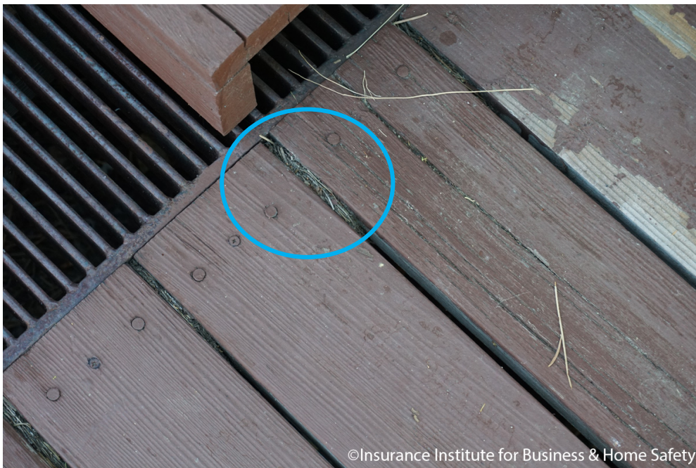
Figure 2. Typical debris accumulation points at deck-to-wall connection (top) and gap between deck boards (bottom).
