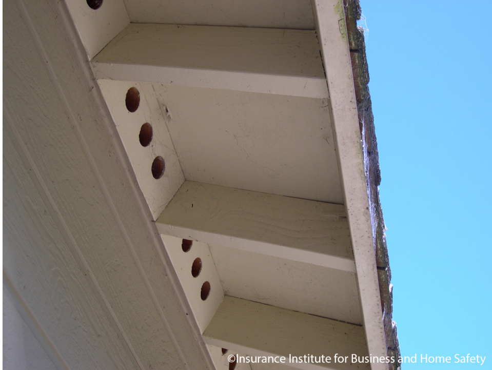
Figure 1. Vents located in between-rafter blocking in the under-eave area of a building that used open-eave construction.
