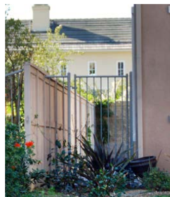
Figure 14. Replace combustible fence sections in the 0–5 ft zone with noncombustible material. Photograph by Stephen Quarles.
