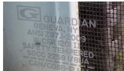
Figure 23. Example of etched label found on tempered glass windows. This is typically found in the bottom corner of the window glass.
