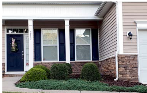
Figure 18. Example of a reentrant corner with combustible siding, windows, bark mulch, and noncompliant vegetation in the corner, which can make a home more vulnerable to wildfire.
